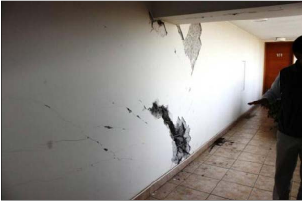
Figure C-3 Damage observed in solid panels at the top and bottom of a stack of openings in the Torre Mayor building in Chillán, Chile following the 2010 Maule earthquake (photo courtesy of EERI Chile earthquake reconnaissance team).
