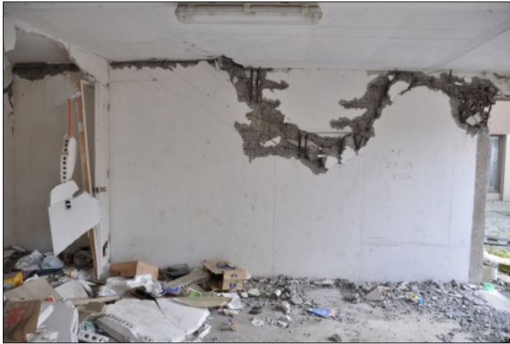
Figure 4-10 Photographs of the damaged section illustrated in Figure 4-9 at wall discontinuity in Plaza del Rio Building A (photos courtesy of Jack Moehle).
