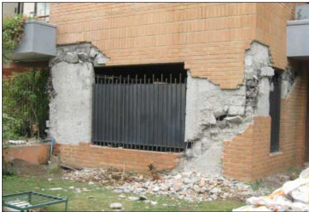
Figure 4-4 Earthquake damage photographs illustrating a geometric wall discontinuity at the Rio Petrohue building, Viña del Mar (photos courtesy of Joseph Maffei).
