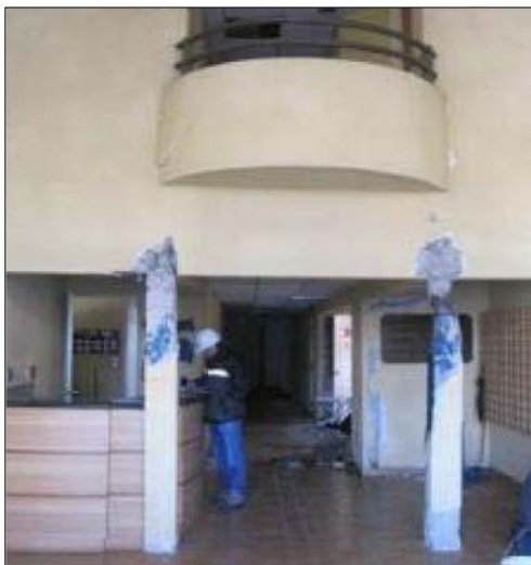
Figure 4-5 Earthquake damage photographs illustrating a geometric discontinuity and geometry change resulting in a wall partially supported on a column in the Centro Mayor building, Concepción (DICTUC, 2010a).
