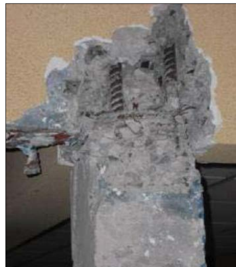
Figure 4-5 Earthquake damage photographs illustrating a geometric discontinuity and geometry change resulting in a wall partially supported on a column in the Centro Mayor building, Concepción (DICTUC, 2010a).
