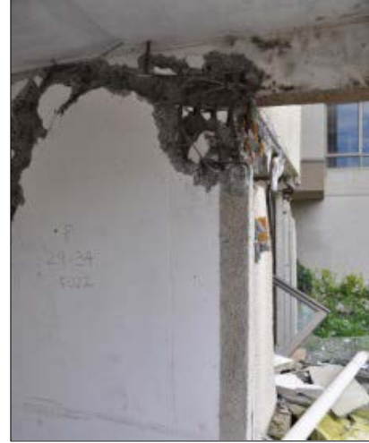
Figure 4-10 Photographs of the damaged section illustrated in Figure 4-9 at wall discontinuity in Plaza del Rio Building A (photos courtesy of Jack Moehle).
