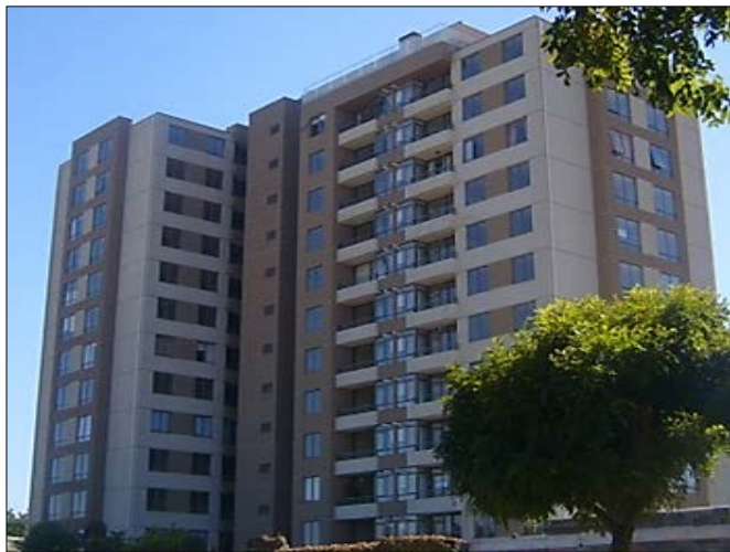
(a) Exterior view of both towers (Cerda, 2011)
