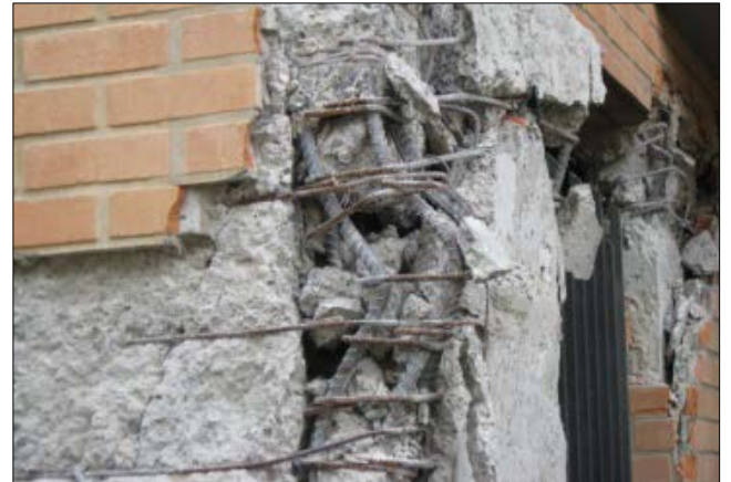
Figure 4-4 Earthquake damage photographs illustrating a geometric wall discontinuity at the Rio Petrohue building, Viña del Mar (photos courtesy of Joseph Maffei).
