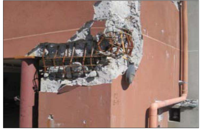
Figure 4-3 Earthquake damage photographs illustrating a geometric wall discontinuity at the Centro Mayor building, Concepción (DICTUC, 2010a).
