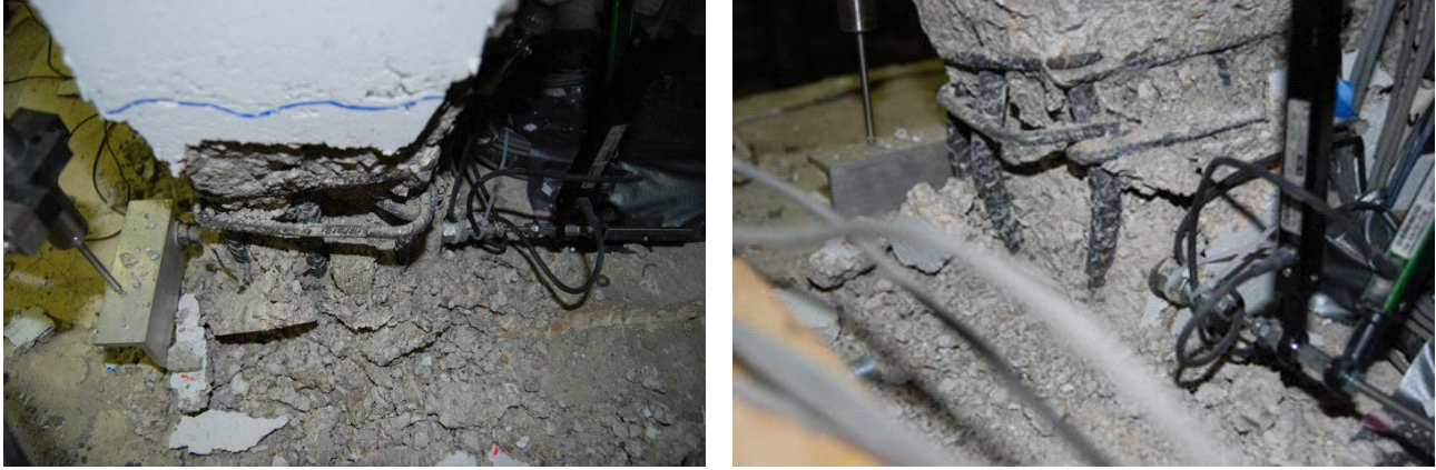
Figure 5-8 Failed toe of specimen PW4 at 0.75% drift (Lowes et al., 2011).
