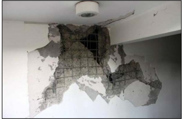
Figure C-3 Damage observed in solid panels at the top and bottom of a stack of openings in the Torre Mayor building in Chillán, Chile following the 2010 Maule earthquake (photo courtesy of EERI Chile earthquake reconnaissance team).
