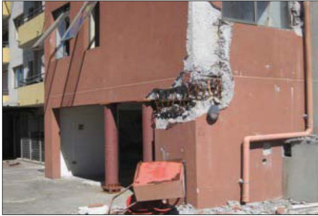
Figure 4-3 Earthquake damage photographs illustrating a geometric wall discontinuity at the Centro Mayor building, Concepción (DICTUC, 2010a).
