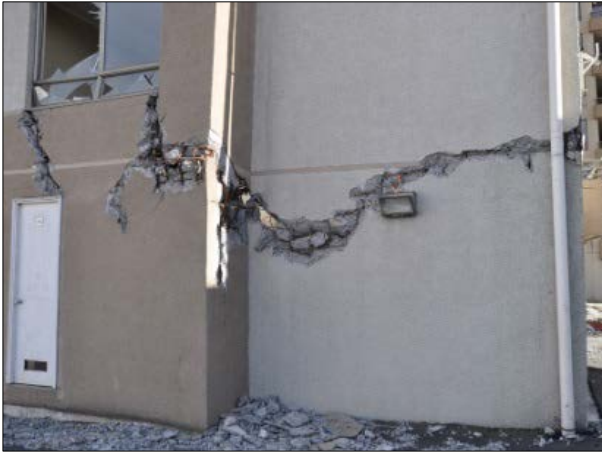
Figure 4-8 Photographs of damage at discontinuities in Z-shaped walls at the south end of Plaza del Rio Building A. Three-dimensional rendering illustrates wall configuration showing that a flange in the second story is not present in the first story. Red regions in the rendering indicate locations of damage (photos courtesy of Jack Moehle).
