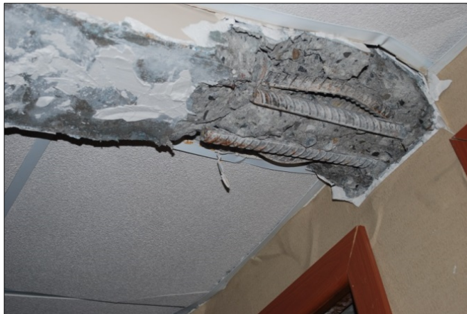
(a) Photo of bar termination (lap splice) in beam hinge region (photo courtesy of Jack Moehle)
